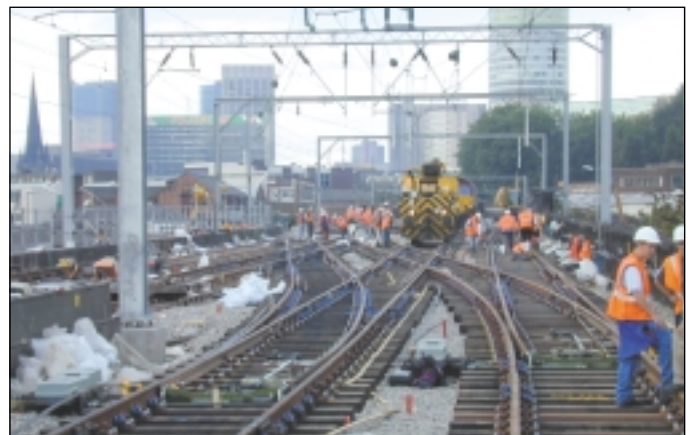
Proof House Junction, Birmingham
