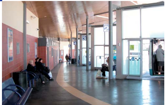
Macclesfield Bus Station – interior
