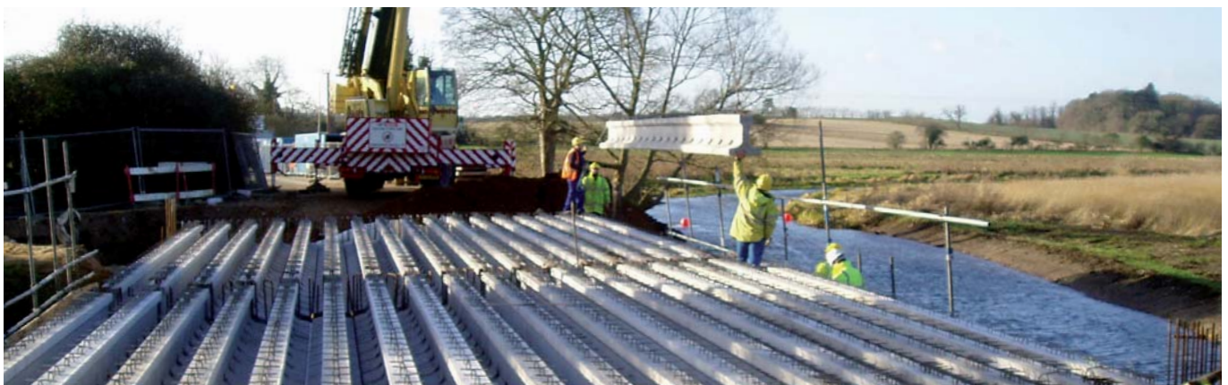
Guist Bridge Development
