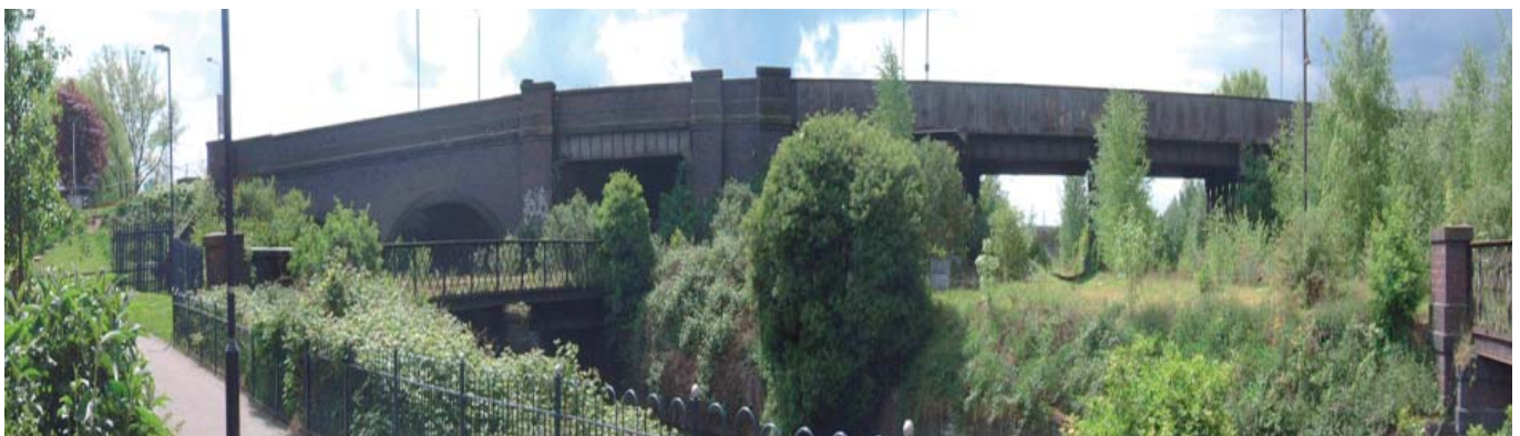
Upperton Road Viaduct: Existing Infrastructure
