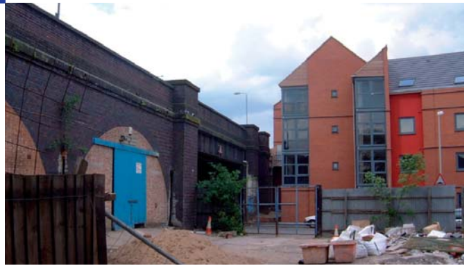
Before: Occupied arches below the viaduct
